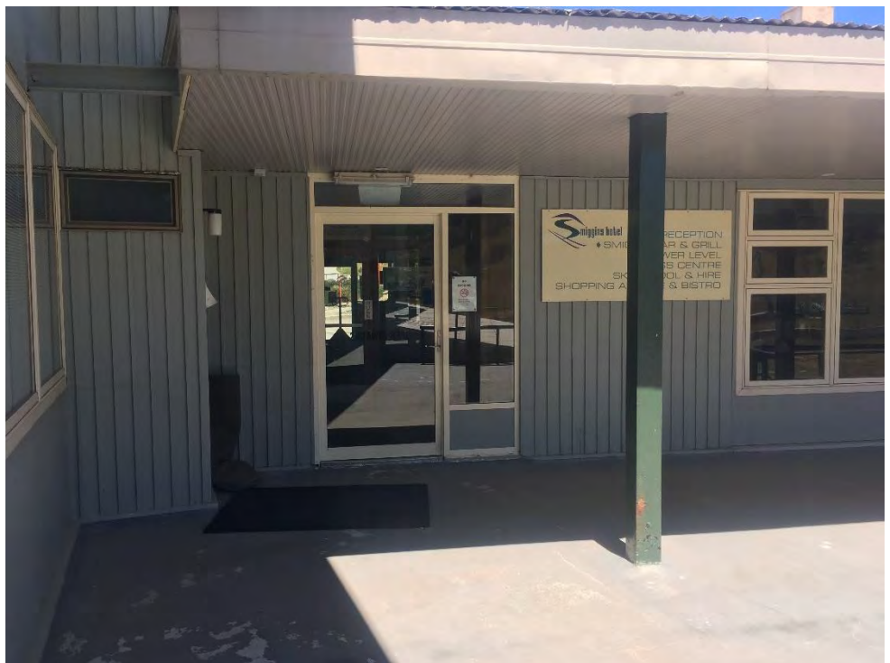
Figure 9: Photo of the location for the air lock addition
