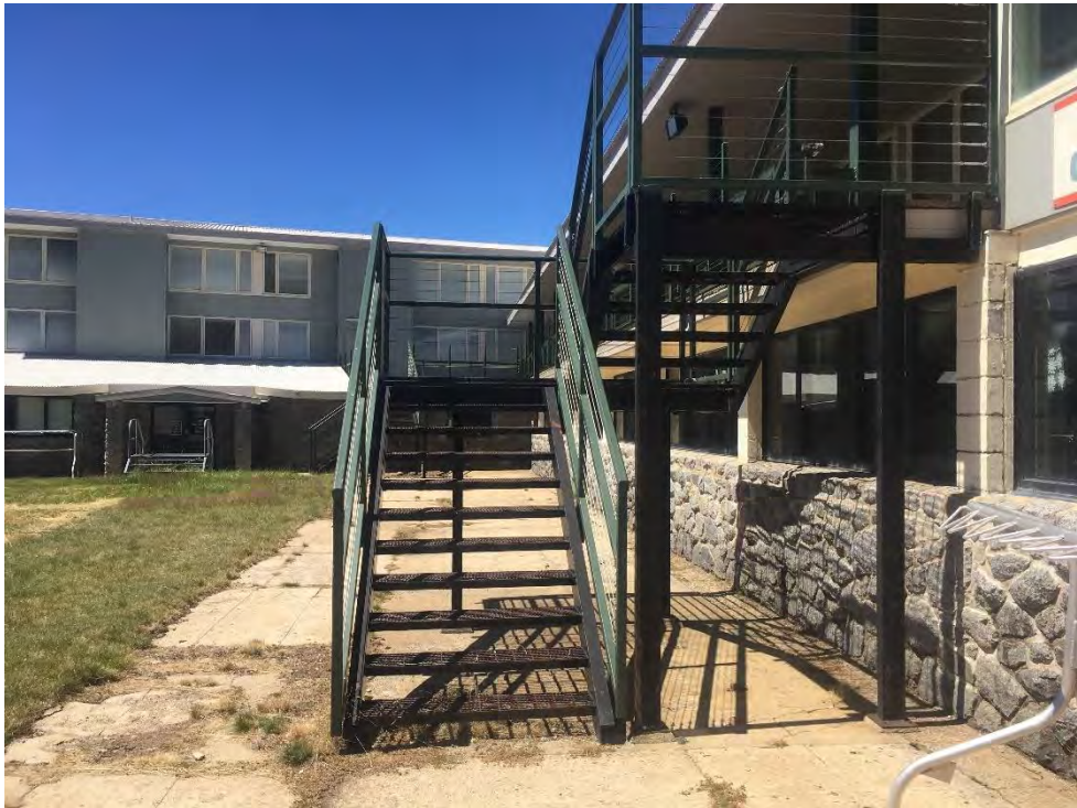
Figure 10: Photo of the staircase to be replaced
